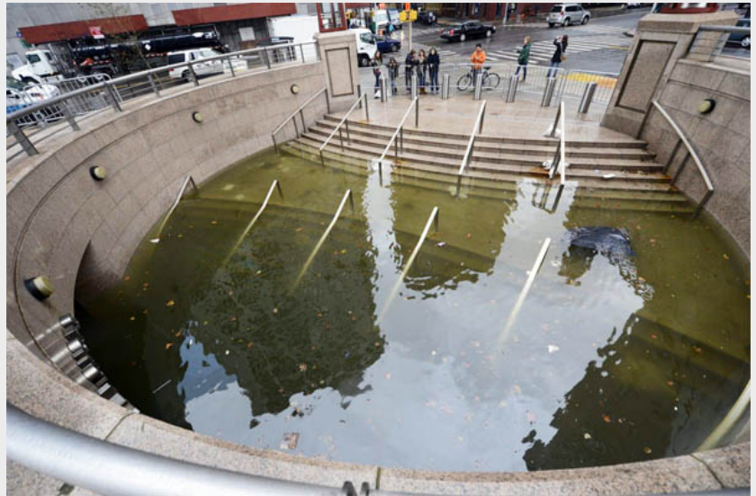
Superstorm Sandy flooded the subways of New York City, an unprecedented event with massive costs. Photo: Timothy A. Cleary, Getty Images
